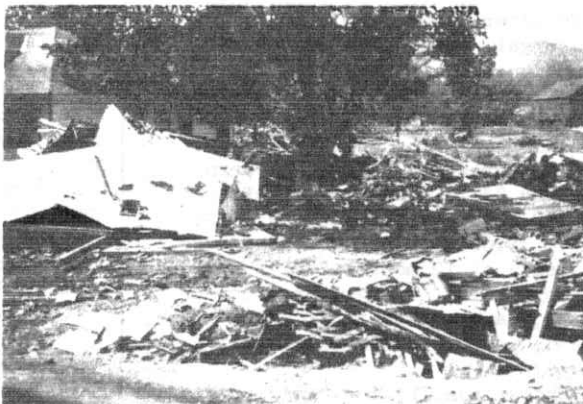
RUBBLE AT THE BRIDGE AT MASSIE'S MILL provides mute testimony of the destruction wrought by the flood waters in the early morning hours of August 20. Countless similar scenes exist.
