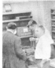
Field Engineer Ralph Abrams "bugs" the gear. . . . .
