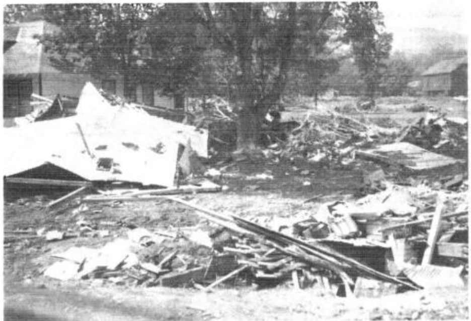
RUBBLE AT THE BRIDGE AT MASSIE'S MILL provides mute testimony of the destruction wrought by the flood waters in the early morning hours of August 20. Countless similar scenes exist.
